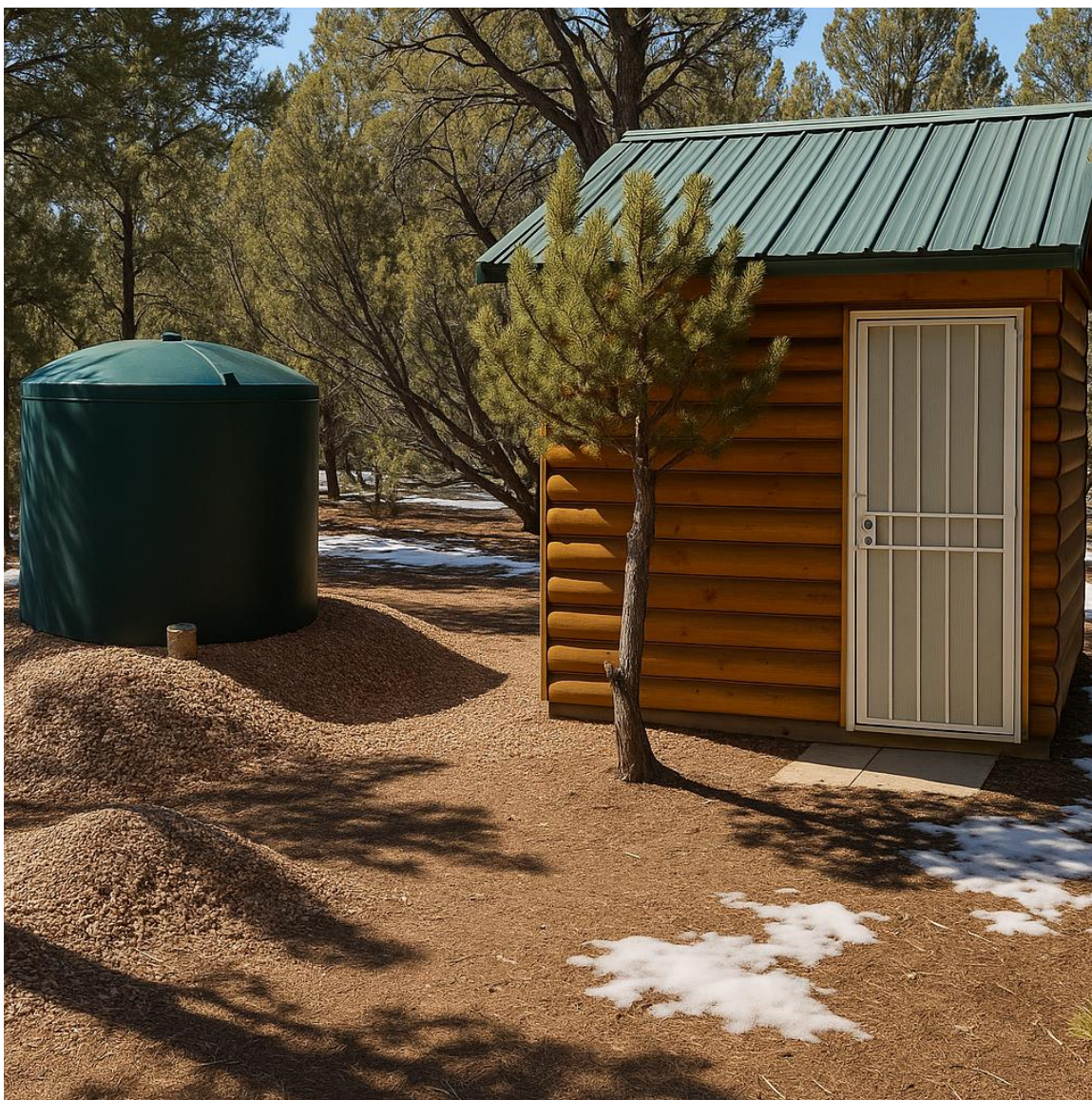
Figure 20 - Above-ground water storage tank and well house. If the well needs to be serviced in the well house, the roof must be removed to allow rig access.
