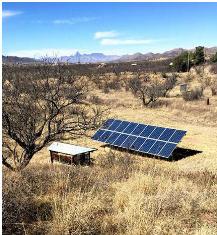
Figure 22 – Solar cells power a domestic well shown in the background.
