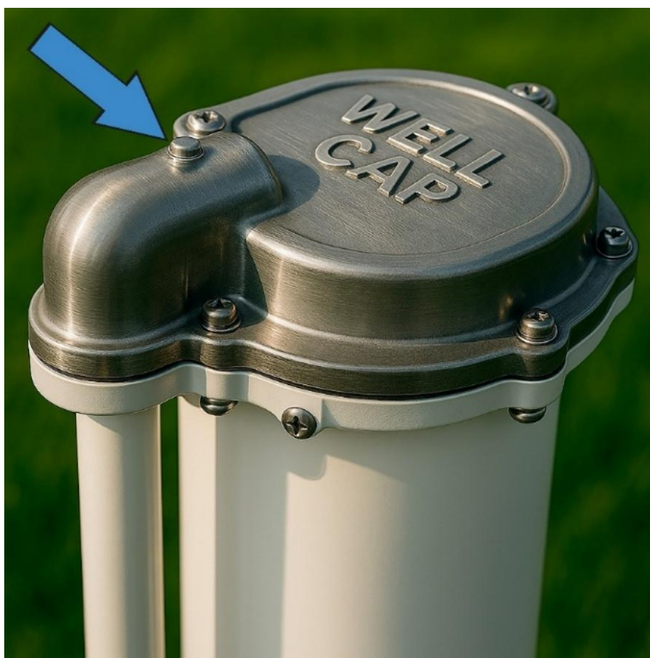
Figure 18 - Example of a well cap made of aluminum. The vent is shown by the arrow.
